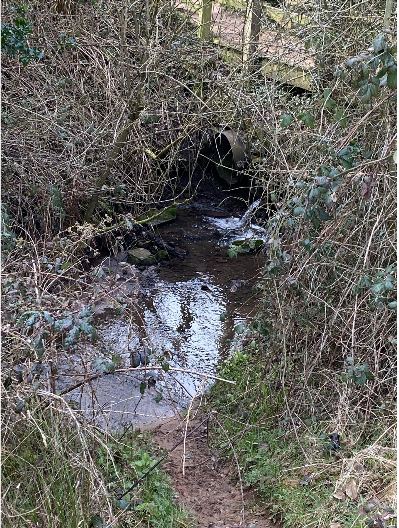
Figure 2.10 View of existing culvert and weir
