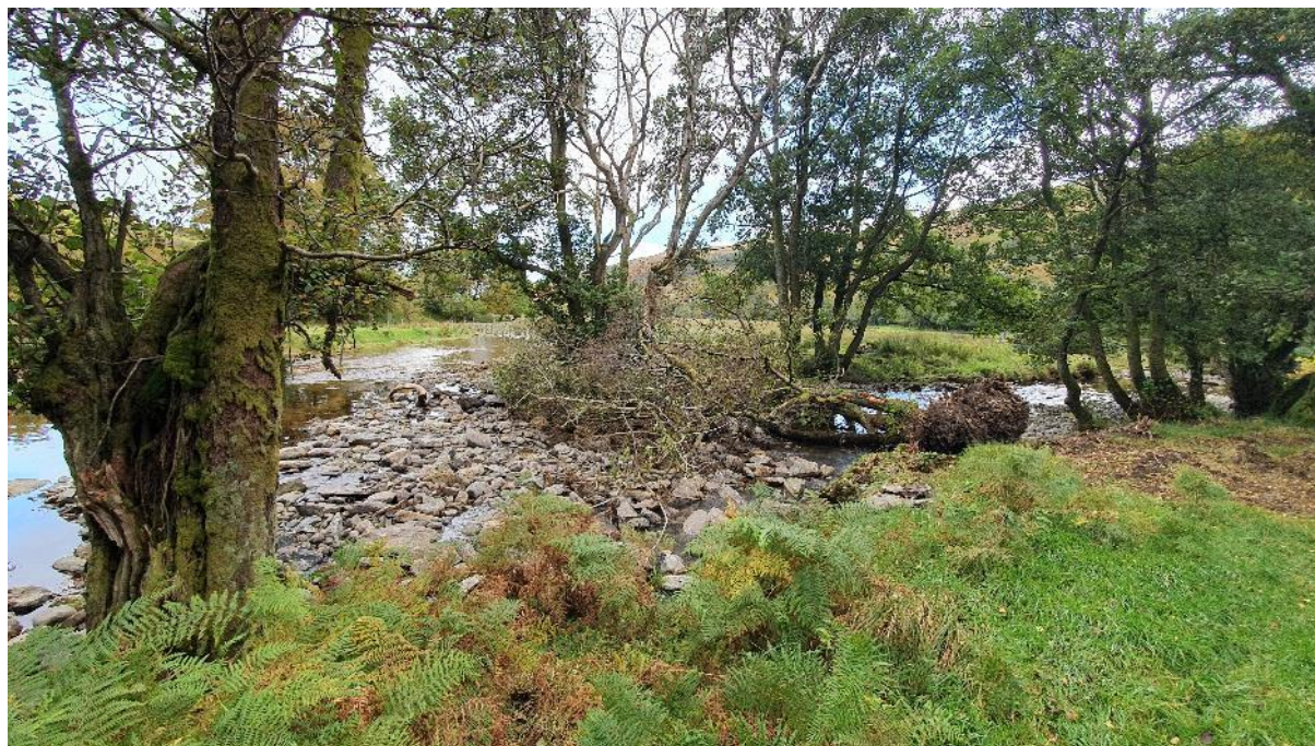
Figure 3.7 Alder pushed over in Swindale Beck to encourage channel avulsion processes.
